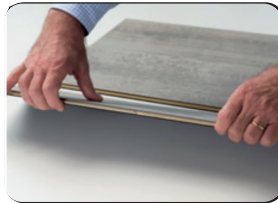
Step 2 Grab the planks with both hands and gently lift at the same time until the planks disengage
