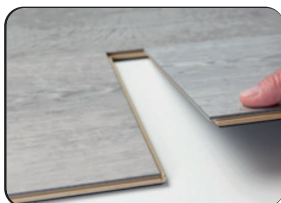
Step 1 Start by engaging the plank on the long side (angle-system)
