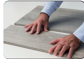
Step 3 Place the planks gently on the floor
