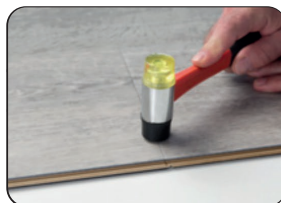
Step 5 Hit gently with a soft-faced hammer on both sides of the short end
