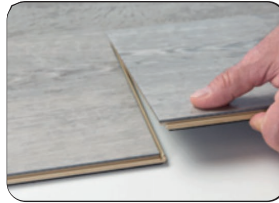
Step 2 Slide the plank until it reaches the short side of the next plank
